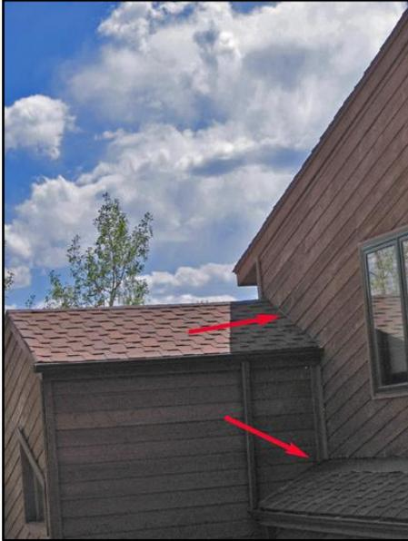
Complex roofs can reduce the protection offered by Class A shingles by allowing firebrands to accumulate at the intersection of the roofing and siding
